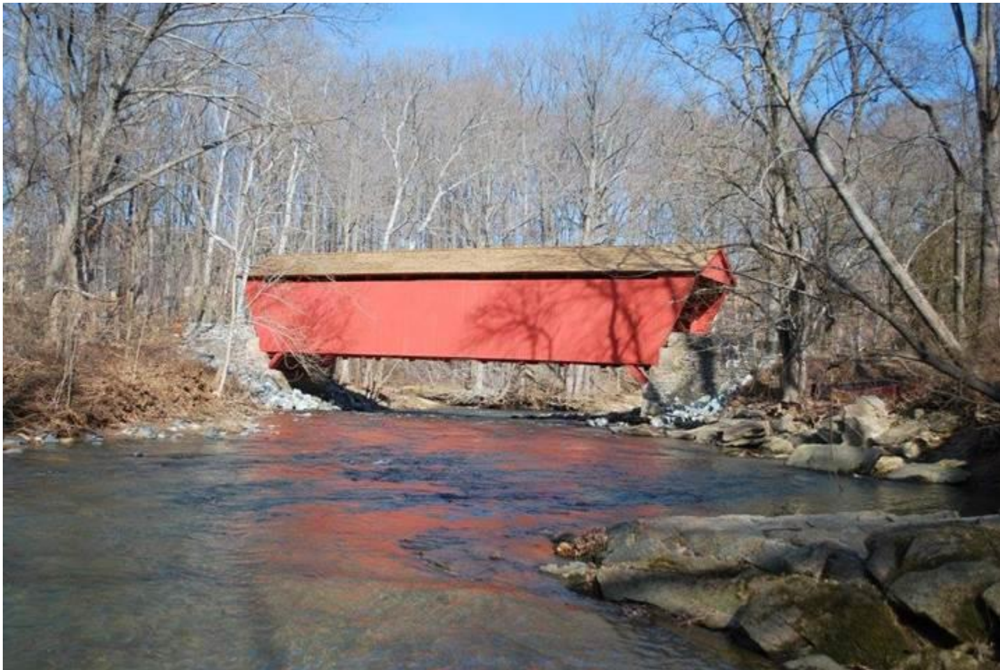
Photo caption: 2016 Preservation Project Awardee: Jericho Covered Bridge Rehabilitation.
